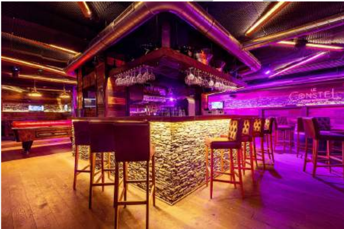
[IMAGE: Pre-fire photograph showing foam-clad ceiling from TripAdvisor (August 2016) promotional photos – Source: TripAdvisor [11]]
